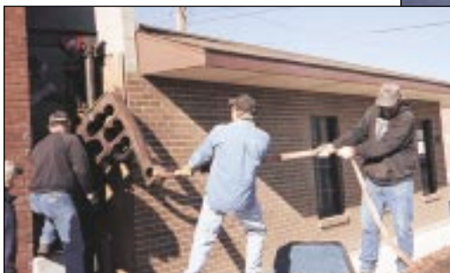
The BCTGM crew pulls the boiler out of the building.
